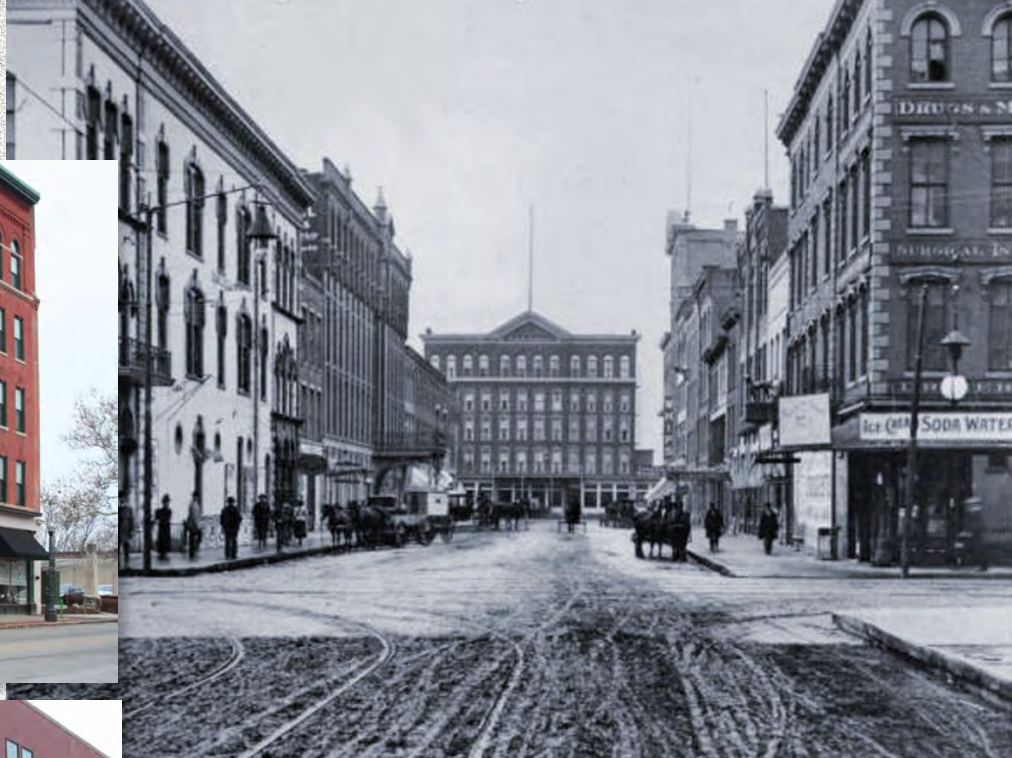
View of the Randall Hotel from Columbia Street c1900
