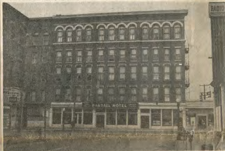
HAD COLORFUL PAST —Once known as Grand Hotel, with no drinking or dancing, the Randall Hotel in its day sheltered VIPs from Benjamin Harrison to Buffalo Bill. It was theatrical headquarters, too during the heyday of Colerick Hall. The building, which marked the western terminus of Columbia Street, was razed in 1965.—Photo by Sid Pepe.
